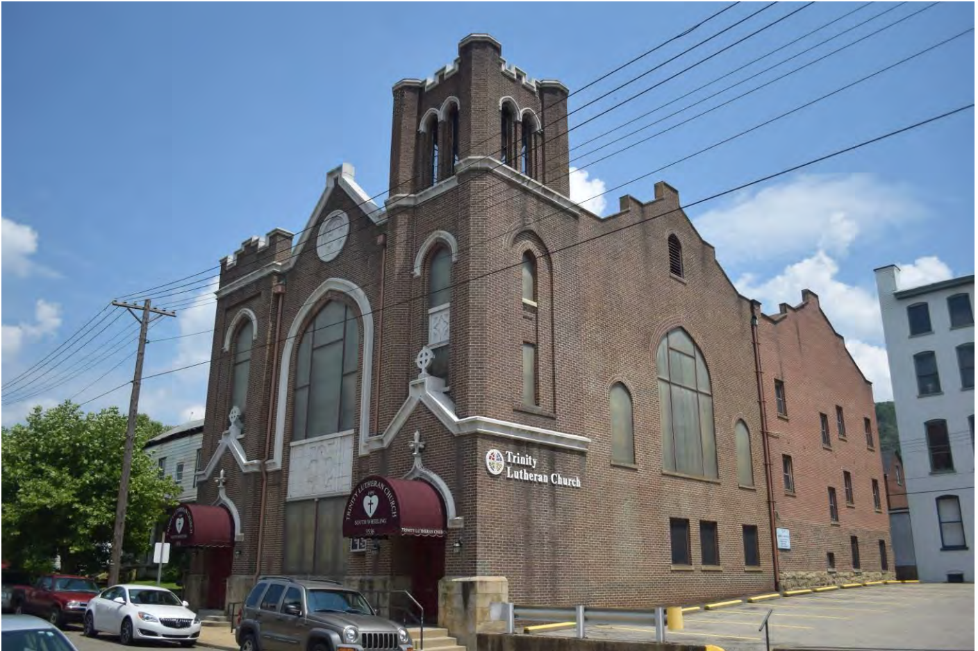
Photo 15. Trinity Evangelical Lutheran Church, 3536 Eoff Street, looking northeast. (R#132)
