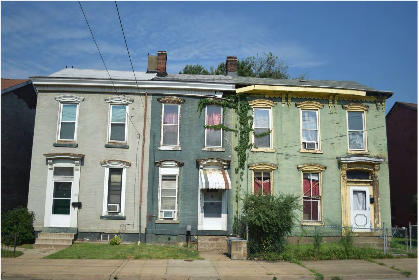
Photo 41. Italianate row houses, 3125-3133 Jacob Street, looking west. (R#113-115)
