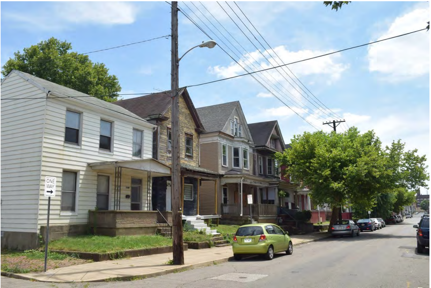
Photo 30. Streetscape, northern end of 3500 block of Eoff Street, east side, looking south.
