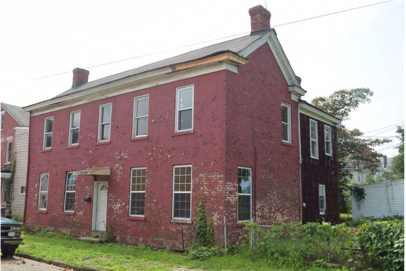
Photo 39. I-house, 6 38 th Street, looking southeast. (R#199)
