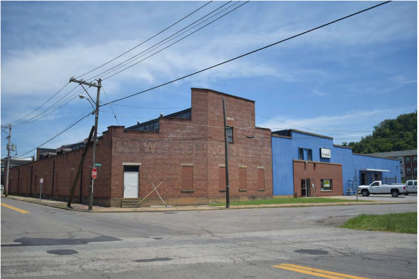
Photo 2. Wheeling Tile Plant 2, 3150 Jacob Street, looking northeast. (R#22)
