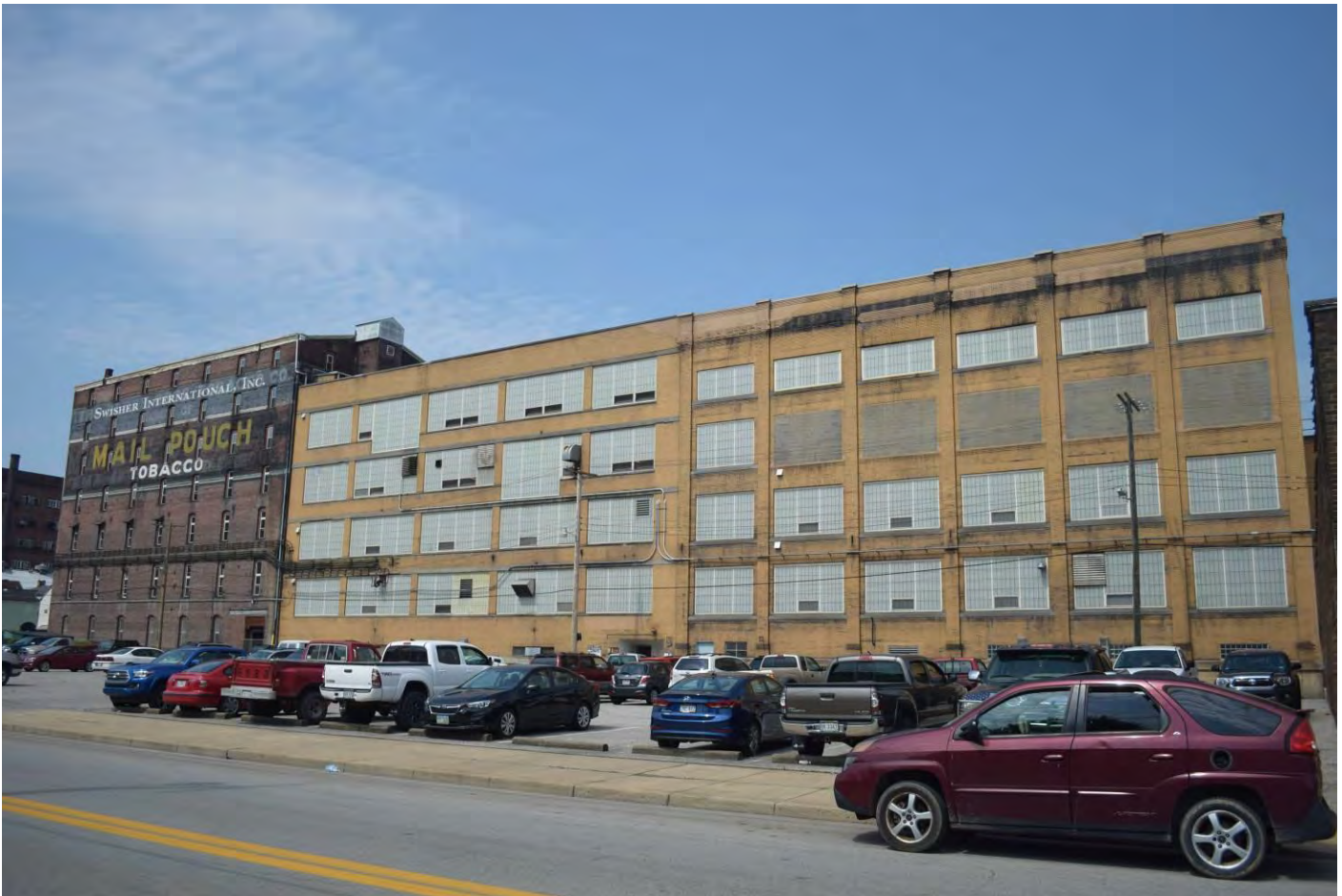
Photo 11. Bloch Brothers Tobacco, 3900 Water Street, looking southwest. (R#277 left, R#278 right)
