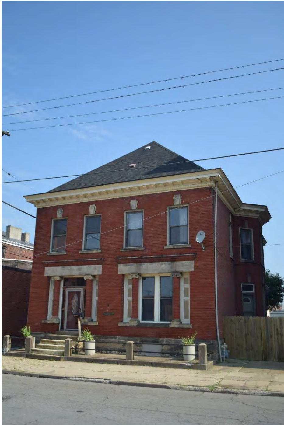
Photo 48. Neoclassical house, 49 36 th Street, looking north. (R#169)
