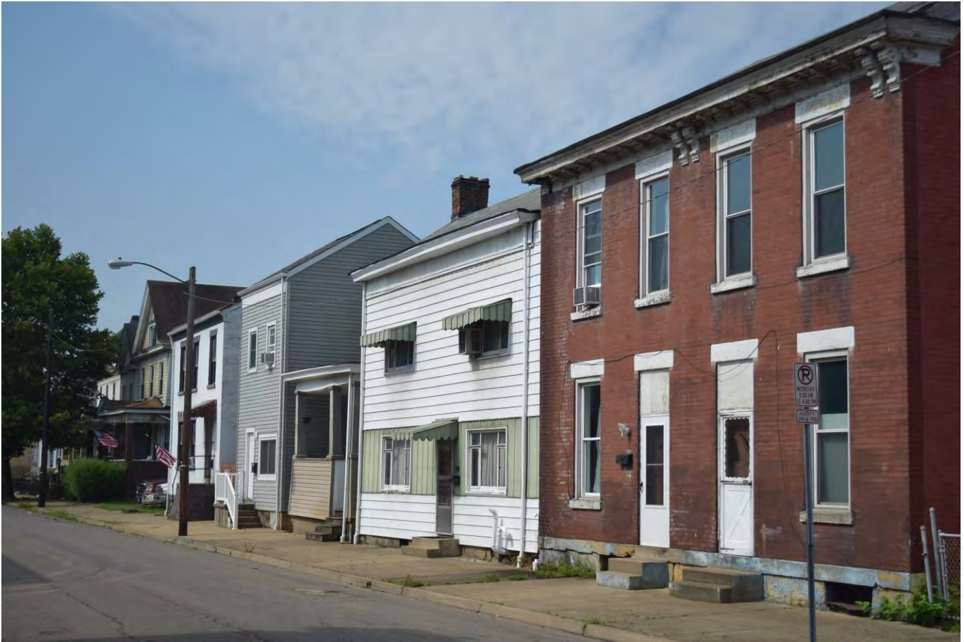
Photo 36. Streetscape, northern end of 3800 block of Eoff Street, west side, looking south.
