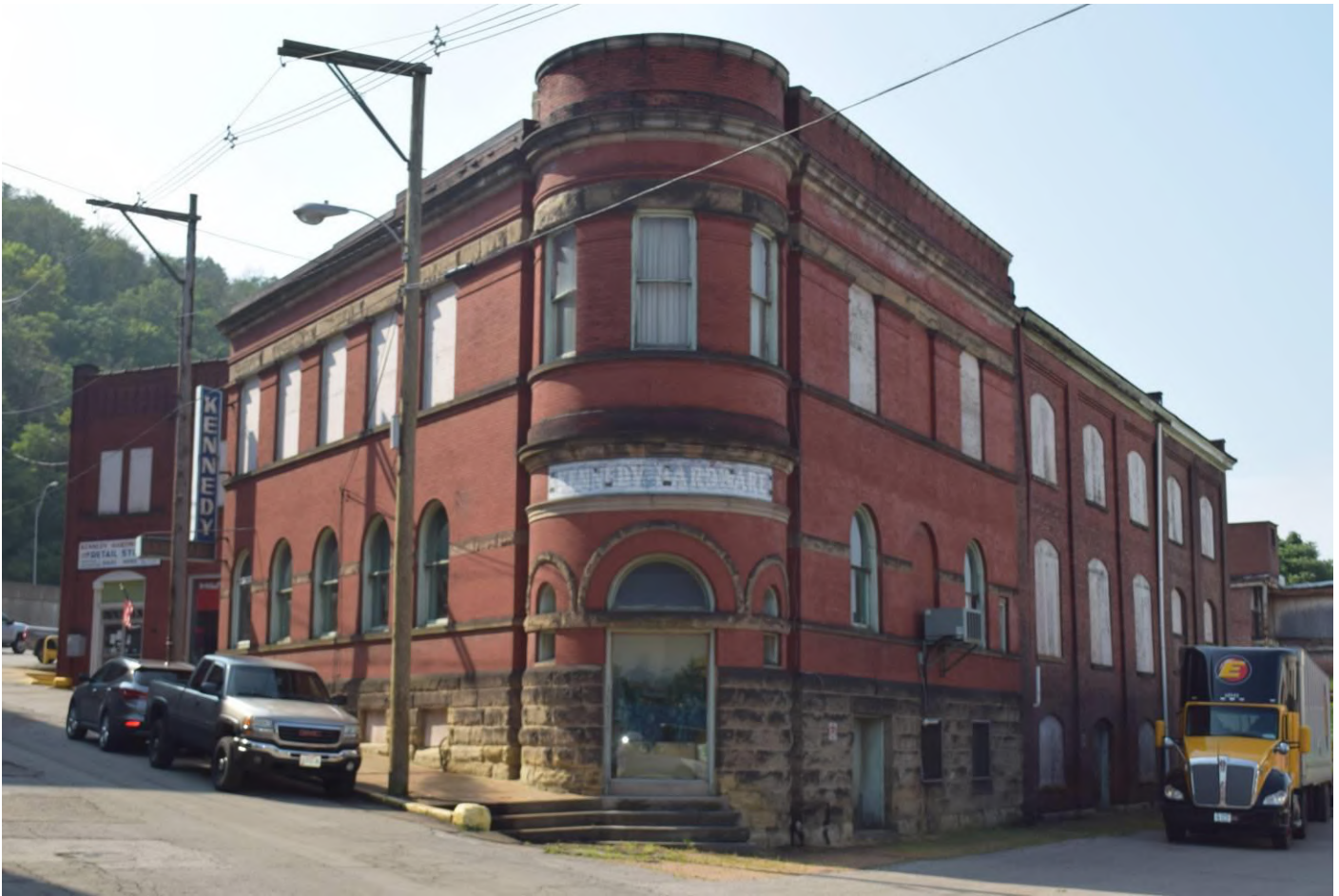
Photo 5. Schmulbach Brewery, Office and Bottling House, 3300 McColloch Street, looking southeast. (R#47, R#46)
