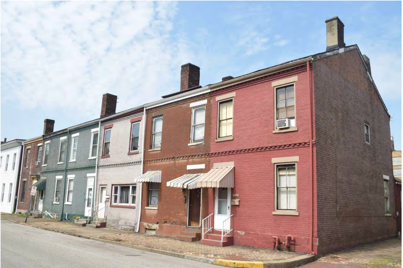
Photo 40. Row houses, 3900 block of Wood Street, west side, looking southwest. (R#312-314, R#316-318)
