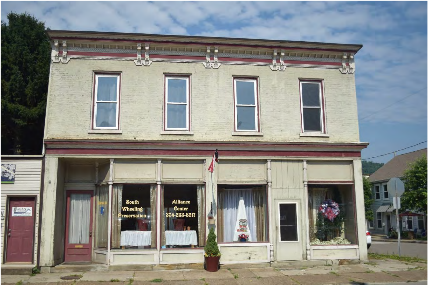
Photo 23. Storefront with residence at upper story, 3501 Jacob Street, looking northwest. (R#144)
