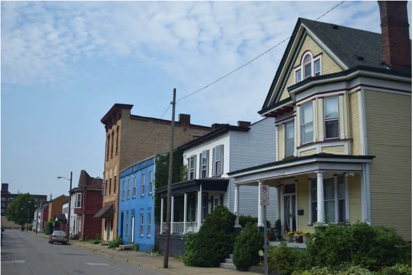
Photo 34. Streetscape, northern end of 3700 block of Eoff Street, west side, looking south.
