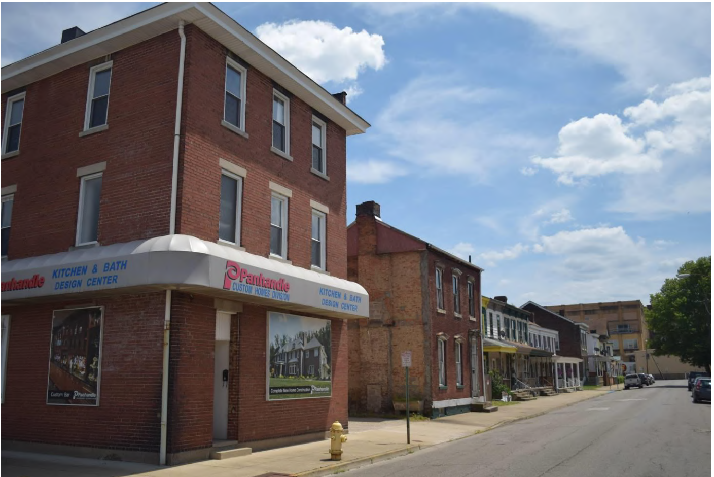
Photo 35. Streetscape, northern end of 3800 block of Eoff Street, east side, looking south.
