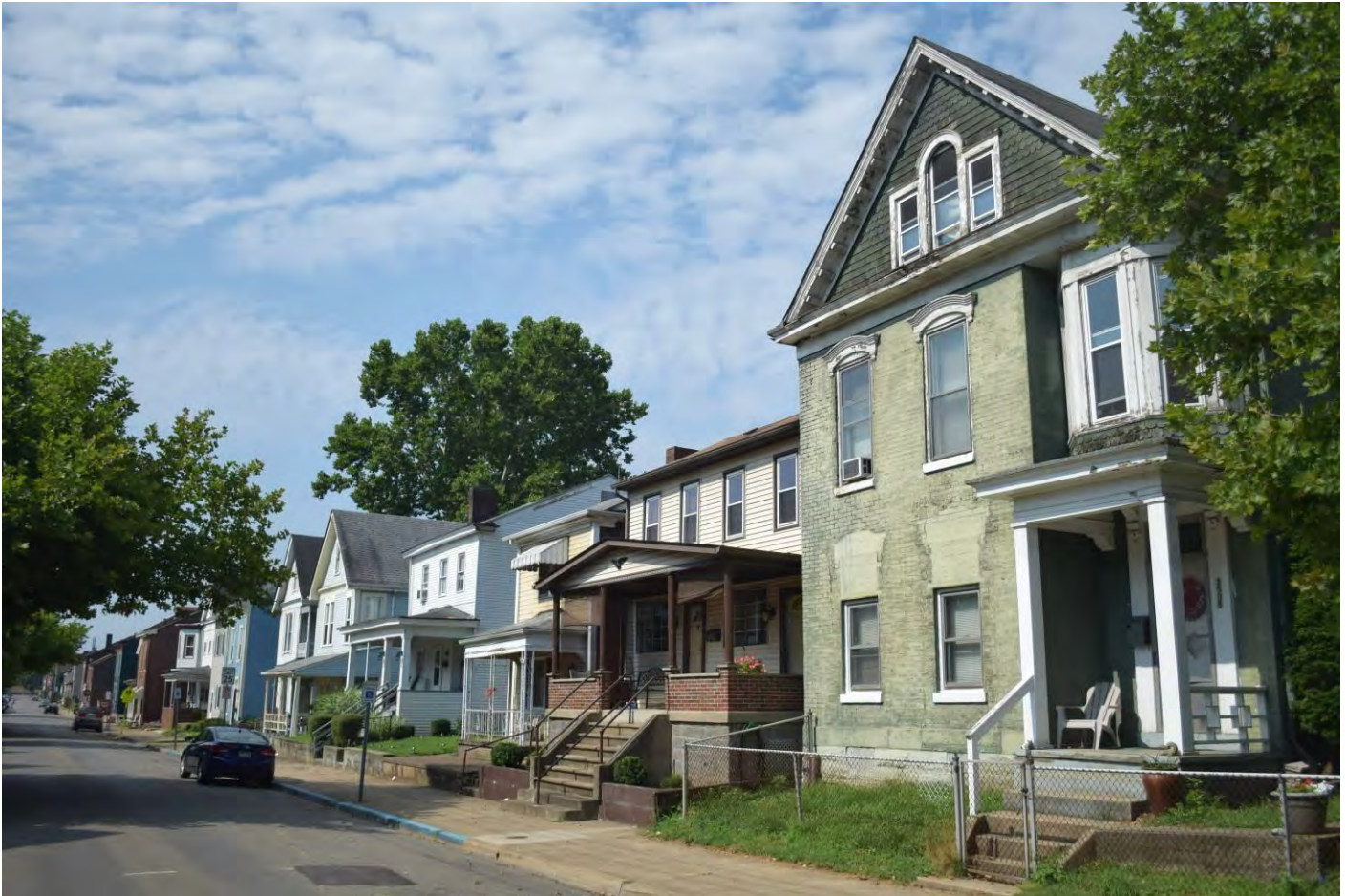
Photo 31. Streetscape, northern end of 3500 block of Eoff Street, west side, looking south.
