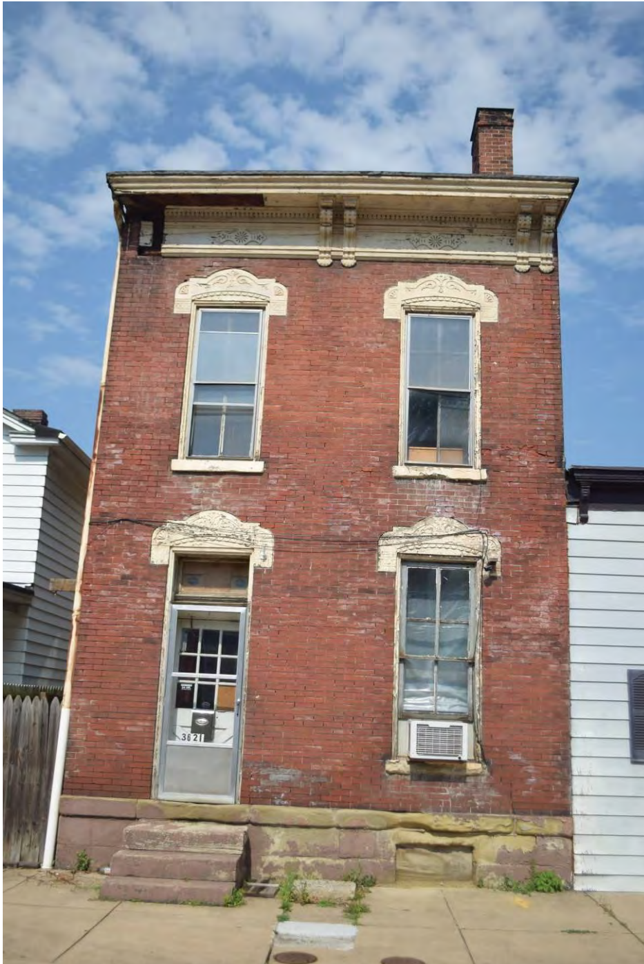
Photo 43. Freestanding Italianate house, 3621 Eoff Street, looking west. (R#109)
