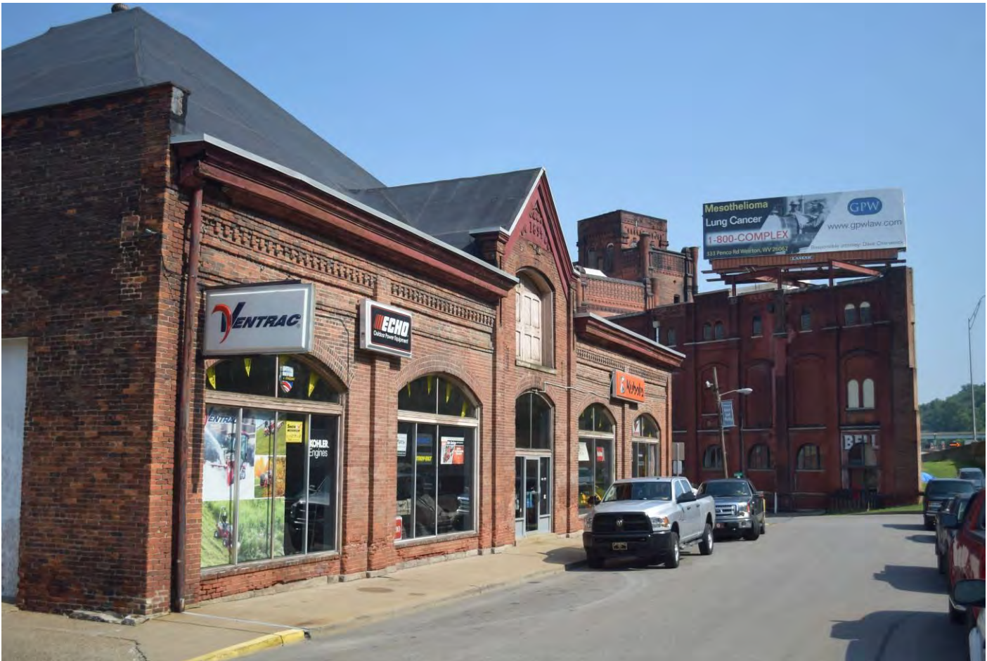
Photo 7. Schmulbach Brewery, Stable, 3305 Wetzel Street, looking northwest. (R#44)
